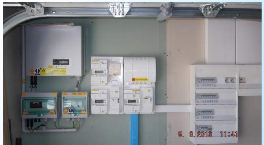
Raccordement monophasé consommation et production
